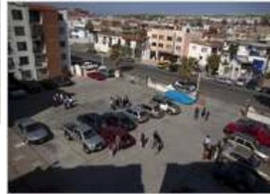
A storage room in a home in El Centro, Calif., after the earthquake.
